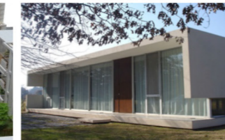
House in Pilar
