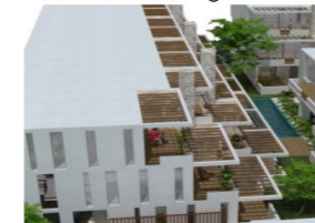
Residential building in Pilar
